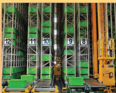
▼自動倉庫 Computer Warehousing
